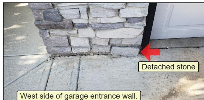
Mortar deterioration
